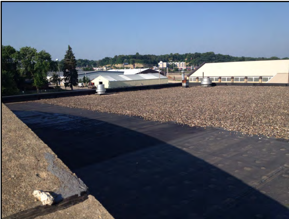
Photo #12: Addition to the west.
