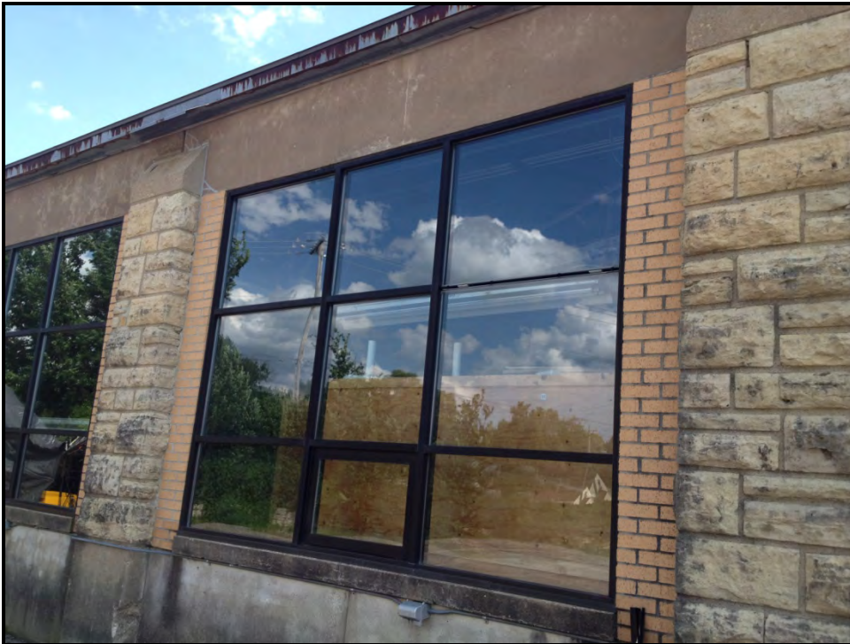
Photo #10: North Elevation – limestone and brick veneer condition.
