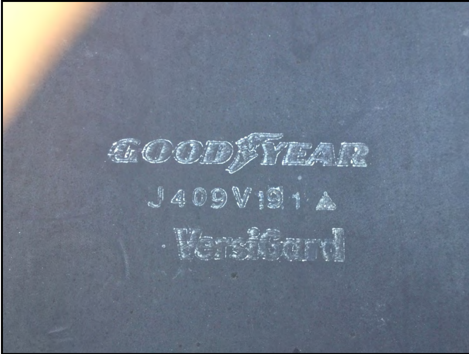
Photo #9: Roof EPDM identification number.
