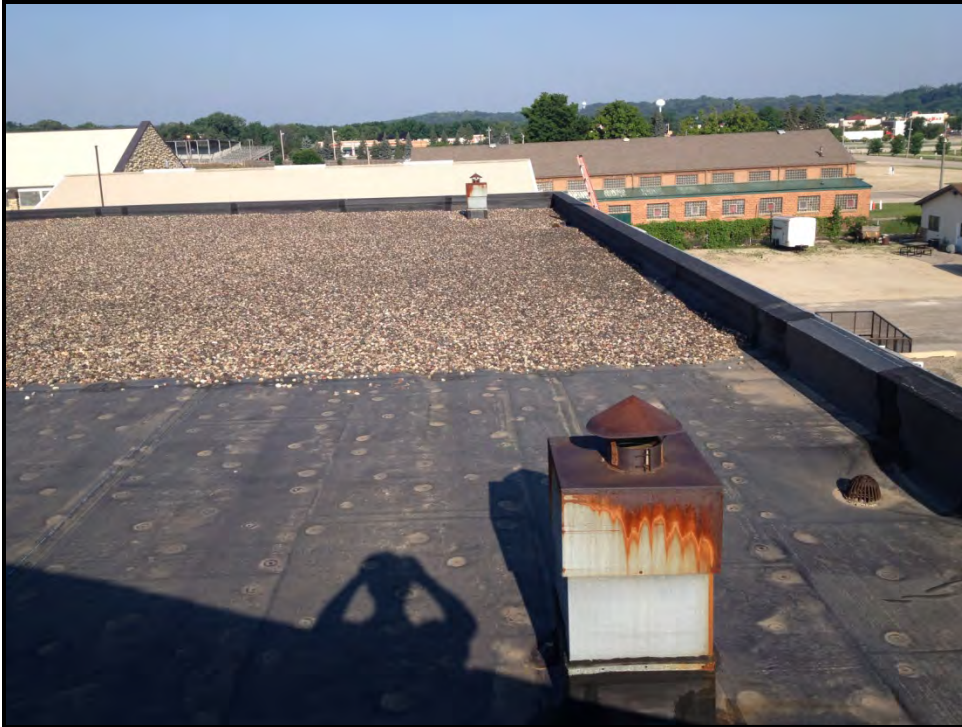
Photo #11: Addition to the west.
