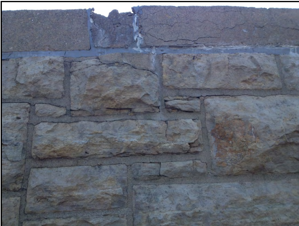
Photo #16: East parapet wall limestone condition.
