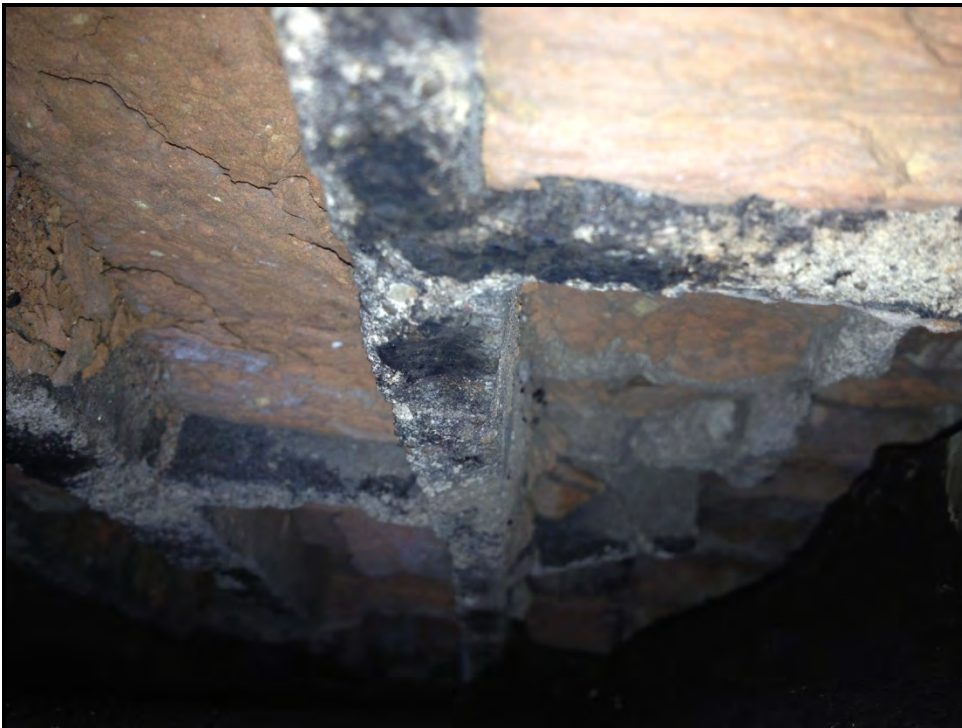
Photo #8: East wall parapet condition. EPDM over brick cavity.
