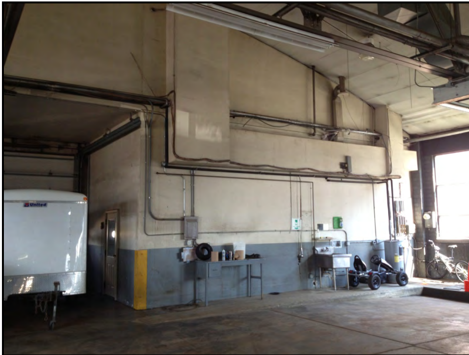
Photo #18: Interior elevation looking east.
