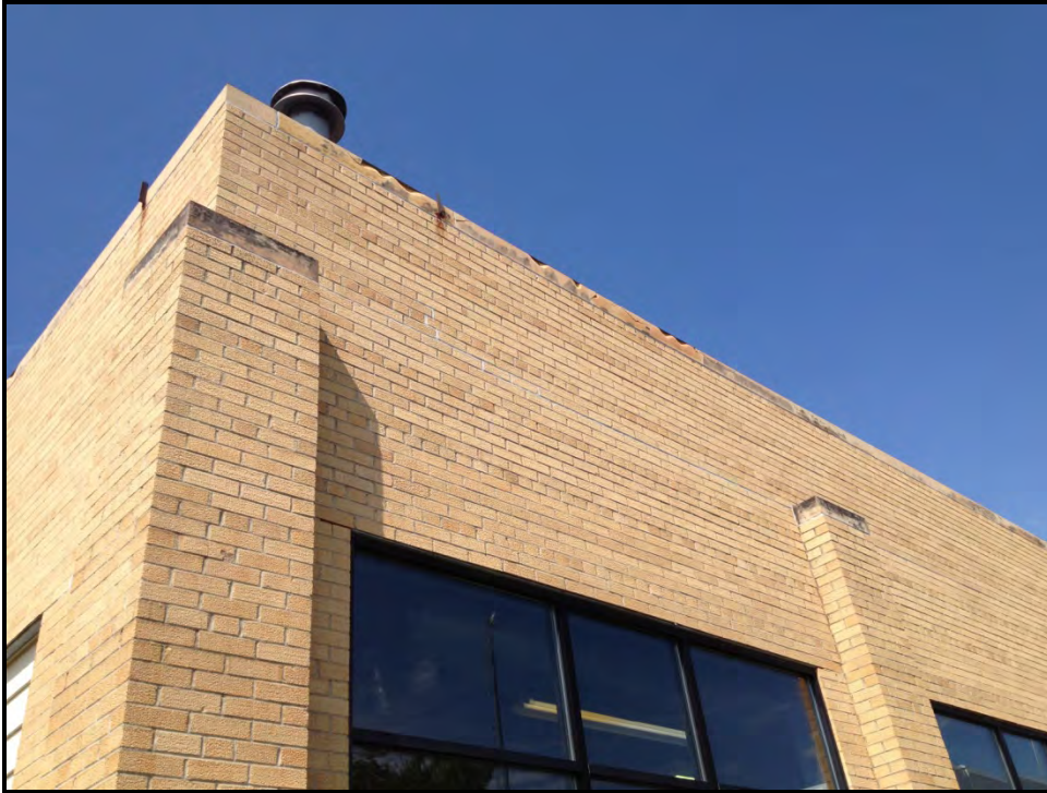
Photo #17: South Elevation – brick veneer and parapet coping condition.
