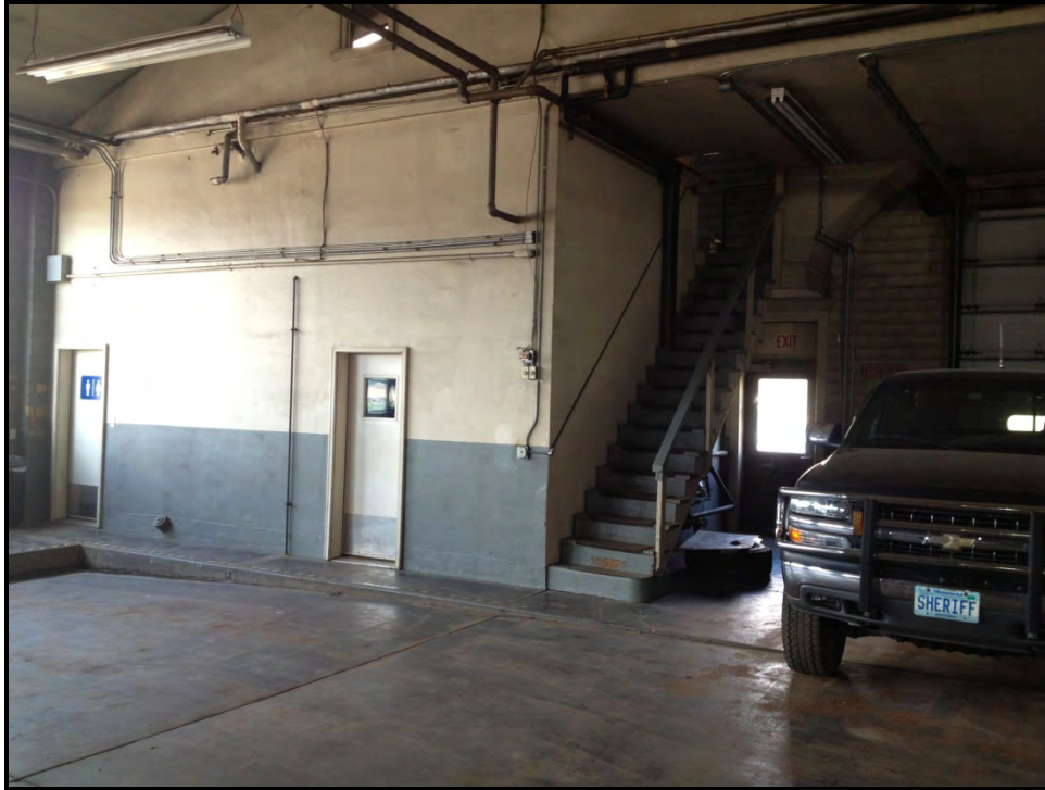
Photo #17: Interior elevation looking east.
