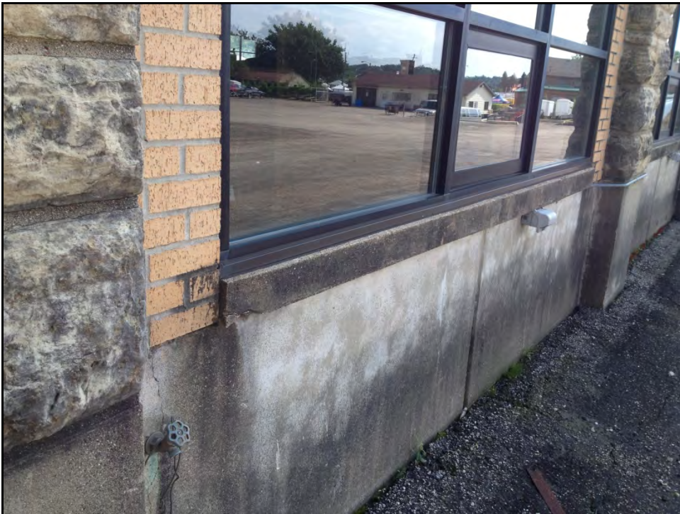
Photo #4: North and South Elevations – window replacements and sill condition.
