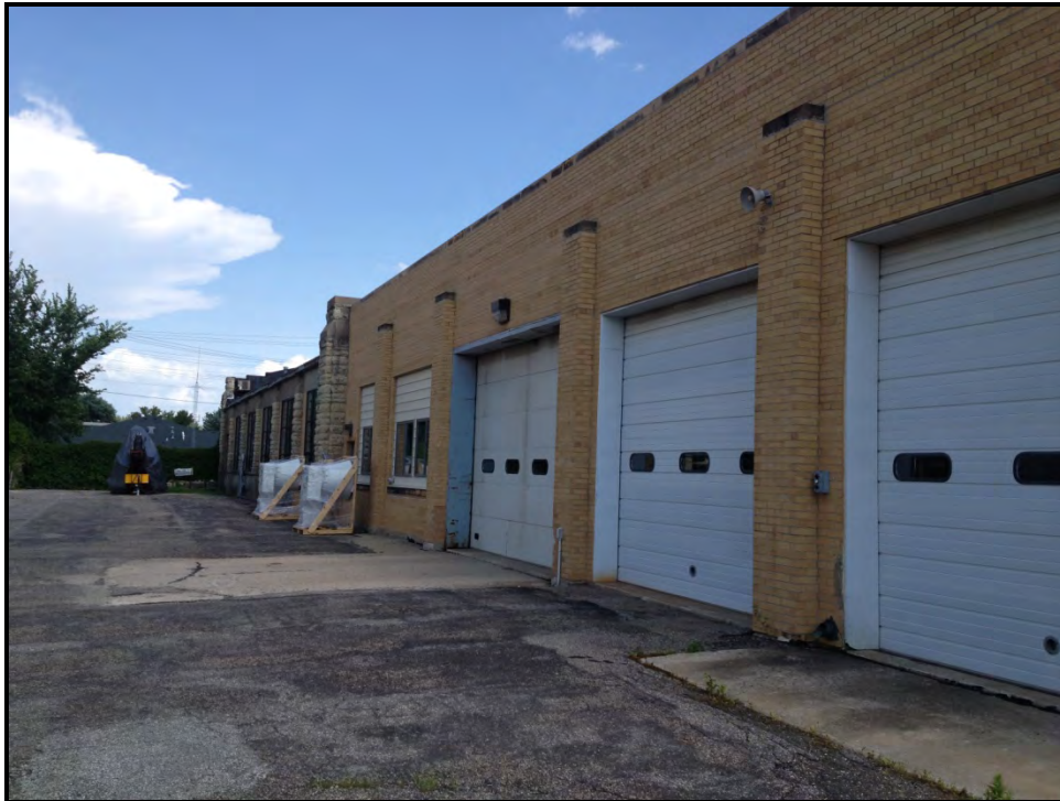
Photo #8: North Elevation – brick veneer and overhead door conditions.
