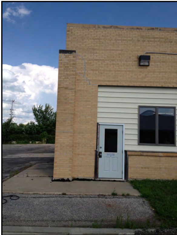
Photo #2: West Elevation – exit door and infill window unit.
