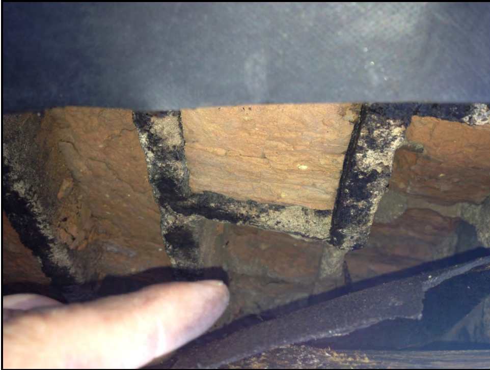
Photo #7: East wall parapet condition. EPDM over brick cavity.
