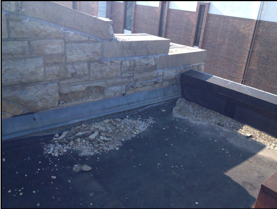
Photo #15: East parapet wall limestone condition.
