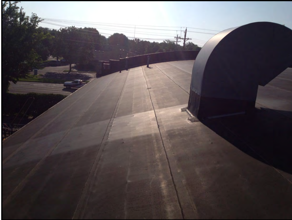
Photo #13: Roof perspective to the east.
