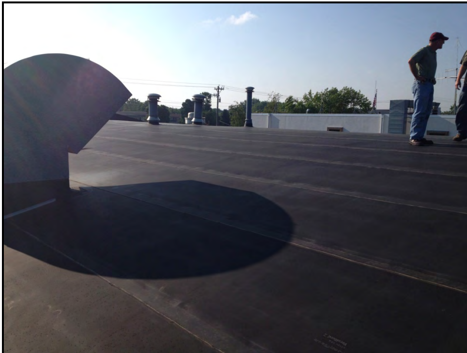
Photo #14: Typical roof installation.
