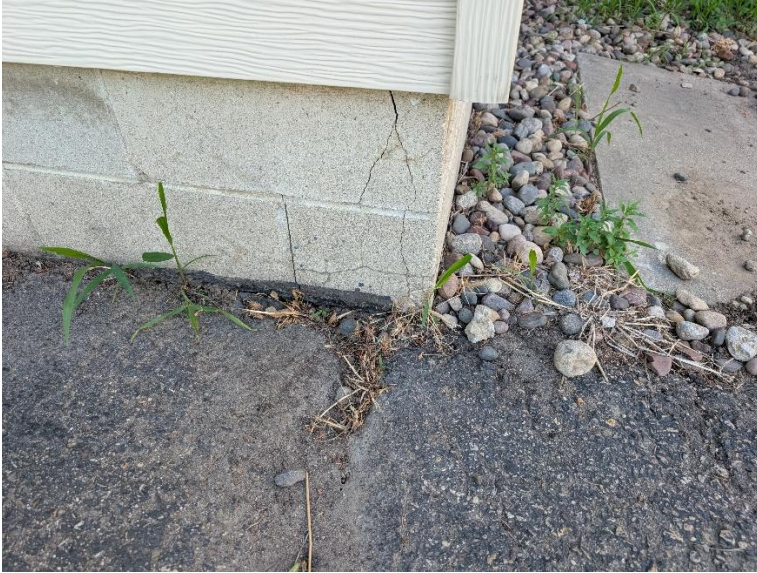
Foundation cracks
